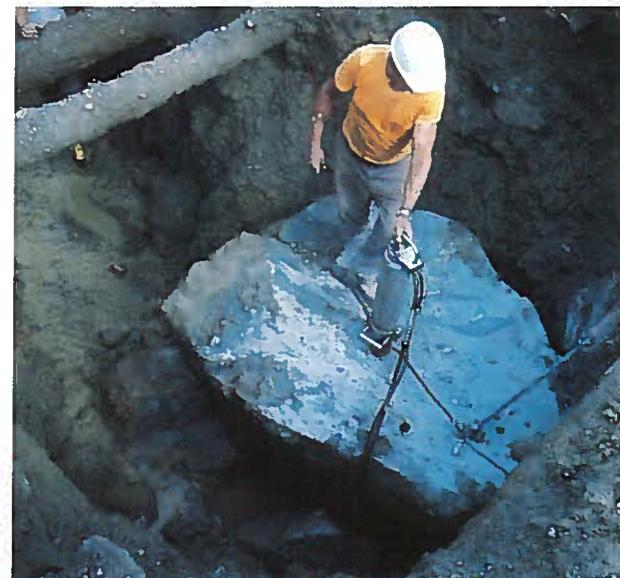
Left, Hydraulic splitter was used to remove ends of overpass supports to form a keyway. The concrete was separated wide enough to cut reinforcing rods using enlarging feathers. Right, Workman carries splitter used to cut 14 ft. tunnel through base of dam for new penstock.
