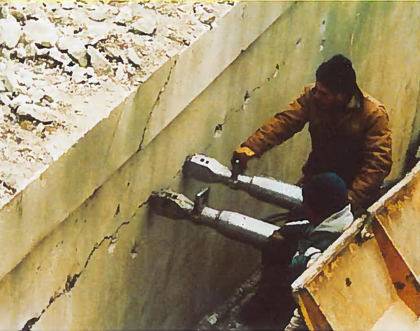
Work crew uses two hydraulic splitters with breaking force of 770 tons to cut two feet off of top of bridge piers. Split was made in less than two minutes along the drill hold line. No impact cracks were left in the remaining lower section to be saved.
