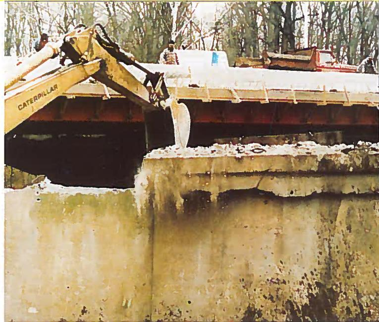
A backhoe quickly topples two ton section off pier top in a few seconds. A new top will be placed on the remaining section to widen the highway from 4 to 6 lanes. Hydraulic splitting method speeds up demolition and reduces costs.
