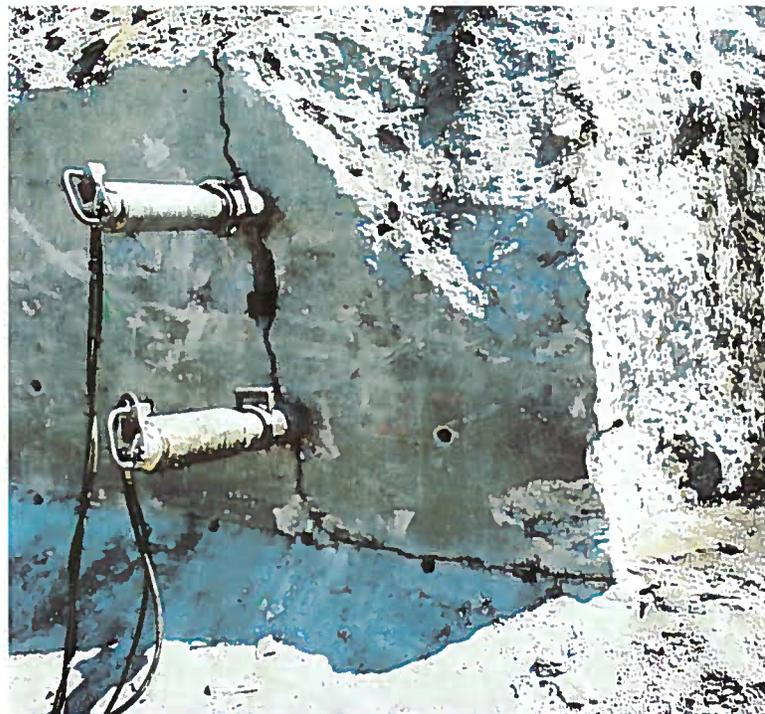
Using two hydraulic splitters, this 8 ft. to 12 ft. thick concrete wall was broken into pieces and removed by a 988 Cat. The contractor speeded up demolition work on this 800 ft. wall many times over other breaking methods.
